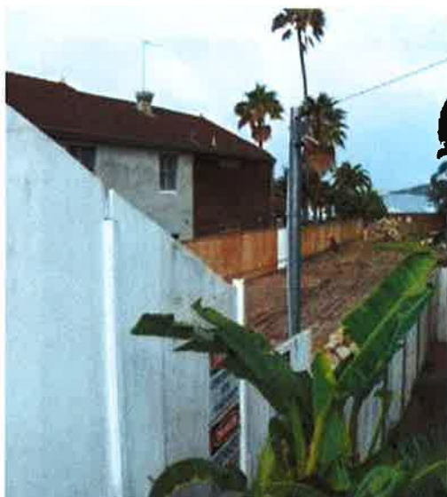
Figure 38 Stuart Street after demolition in 2010.
